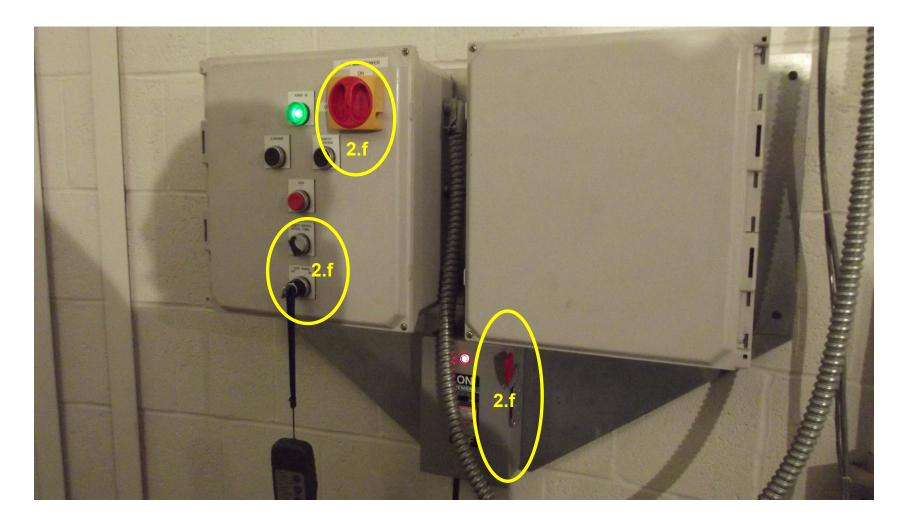
Figure 4: Dome-power connections and switches, which should always be left in the positions indicated.
