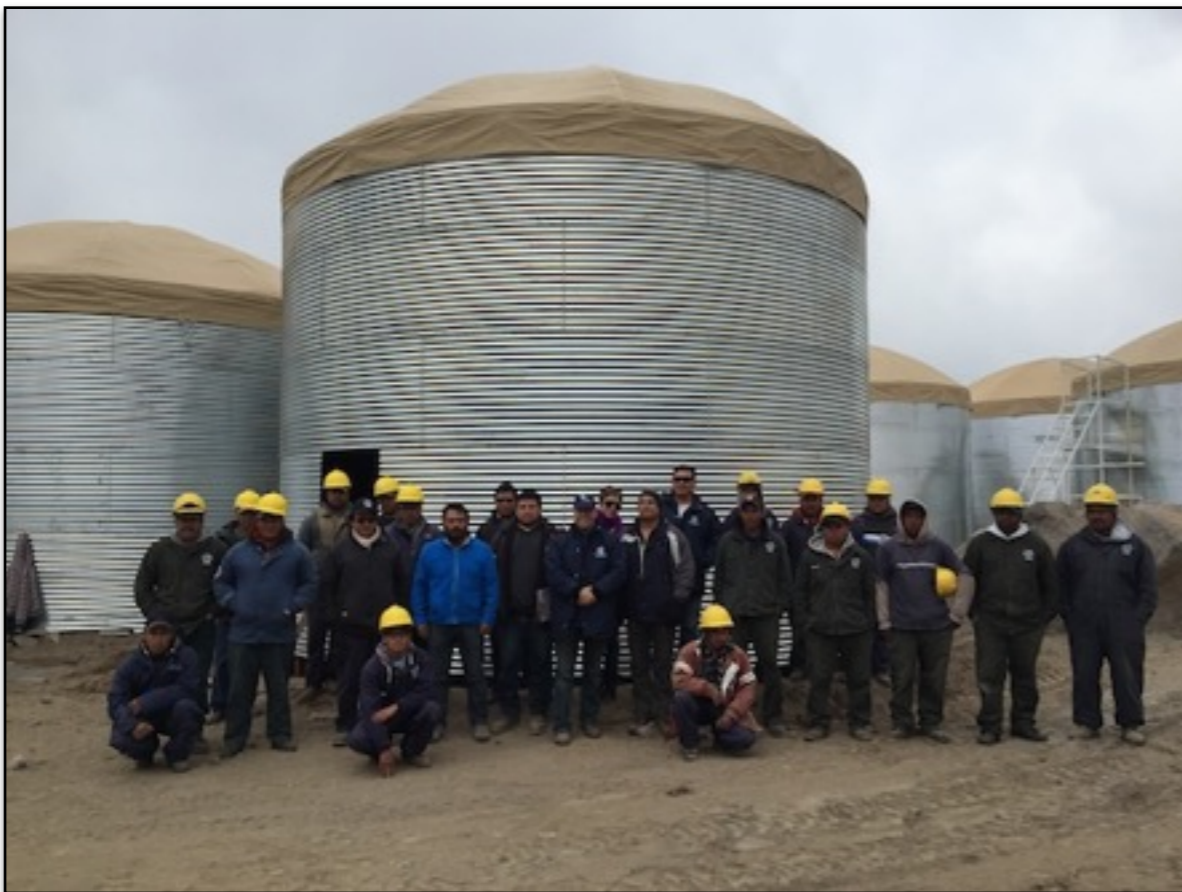
Final tank deployed: December 15, 2014
