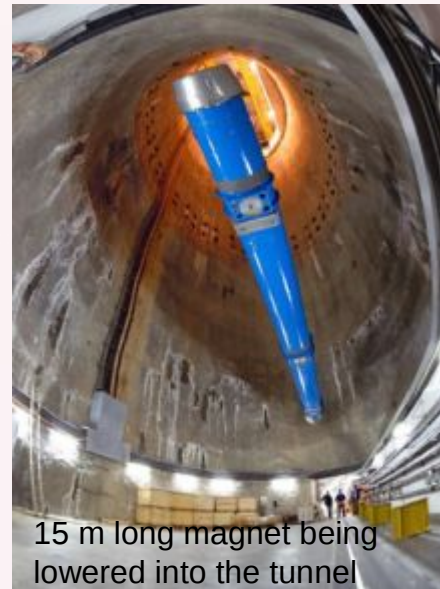
Dipole magnet with the two beampipes
