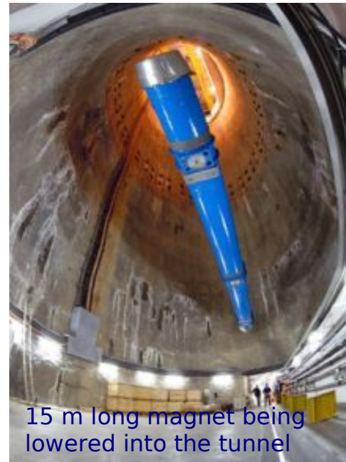
Dipole magnet with the two beampipes
